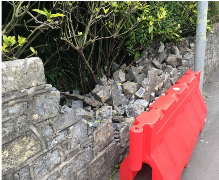
Park Street at St Leonard's junction - October 2022
